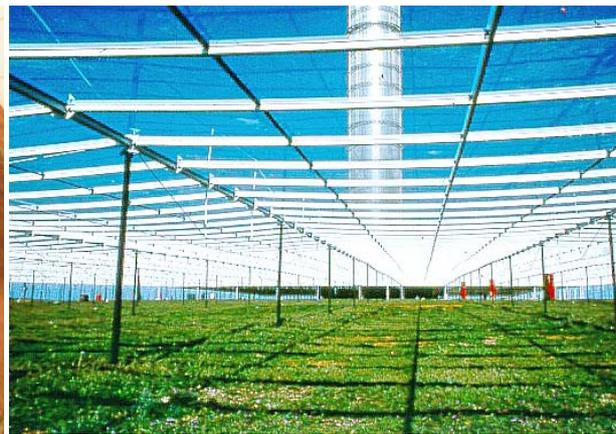
**Figure 8. Glass roof of the prototype plant**
