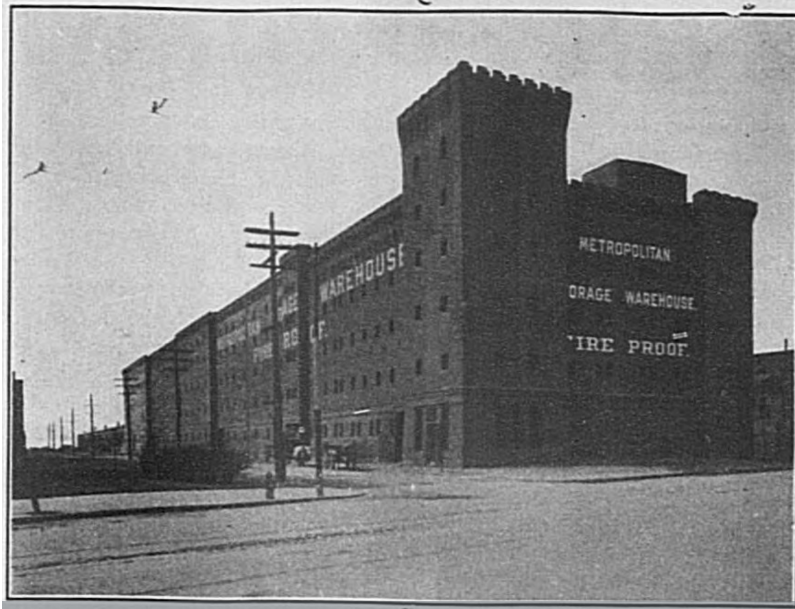
Image of the Metropolitan Storage Warehouse Company, The Cambridge Sentinel , 1920
