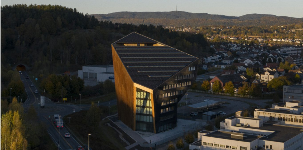
Figure 3: Powerhouse Telemark by Snohetta, 2020, Porsgrunn, Norway (Source: https://snohetta.com/projects/523-powerhouse-telemark-a-sustainable-model-for-the-future-of-workspaces )
