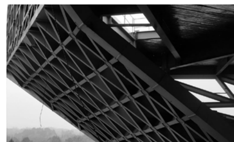
Construction photos, Spring 2022
