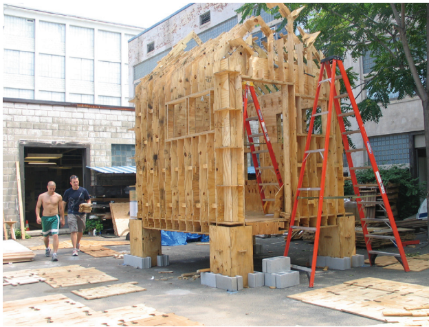
◁ Opening Figure. Hand-guided assembly of interlocking planar elements of an exhibition structure in Sweden. (Credit: All figures by author.)
