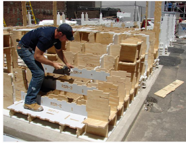
Numbered components support novice assembly
