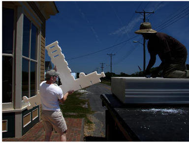
Digital manufacturing in Virginia. Elements were flatpacked for transportation
