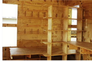
Cabin interior of shelving and desk fabricated after the cabin exterior was assembled
