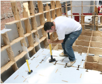
Only four tools were used to assemble the house; Rubber mallets, sledge hammer, clamps, handheld routers
