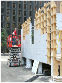
Crane free job site
